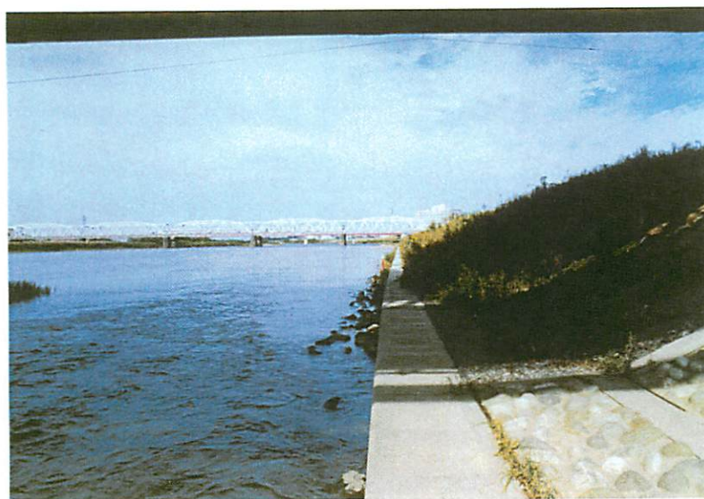
Fig. 8 Bank for low water situated from Jinzu Great Bridge to Railway Bridge on October 7, 2004.
